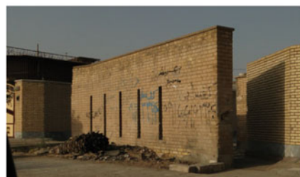
d. Brick screens in labourers' quarters blocking direct view into streets
