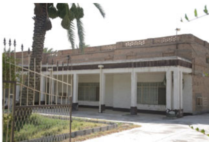
b. Braim: an architecture of brick ornaments and lattices, verandas and ceiling-level ventilation
