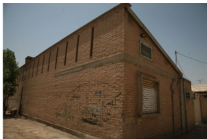
b. Labourers' type with secondary ventilated roof
