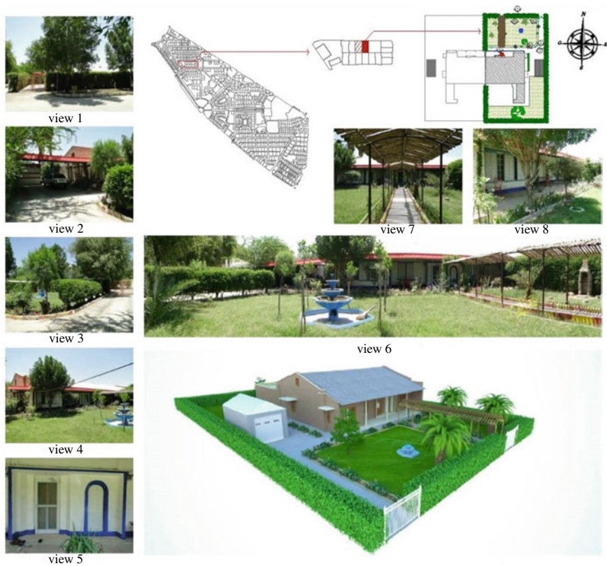
Fig. 12.10 A semi-detached house in Braim with secondary ventilated pitched roof, garage and service block attached to the building. Source Authors
