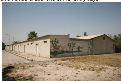
f. Bovardeh; row houses with service blocks facing back street
