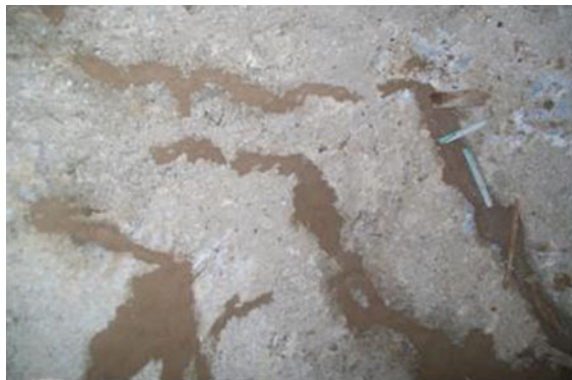
Fig. 10.13 Filling the cracks
