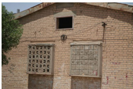
f. Secondary ventilated roof and feature windows in labourers' quarters
