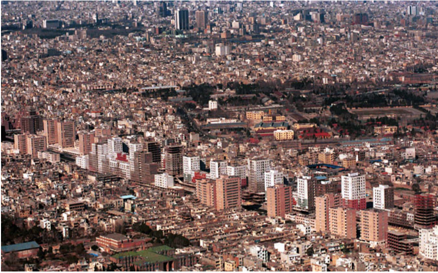
Fig. 5.2 The construction of the edges of the Navvab Highway in Tehran (Andalib and Hajialiakbari 2008, p. 36)
