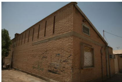
b. Labourers' type with secondary ventilated roof
