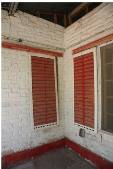
c. Braim; external blinds and ventilated secondary pitched roof
