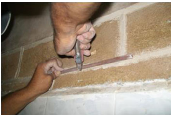
Fig. 10.15 Filling the joints between stones
