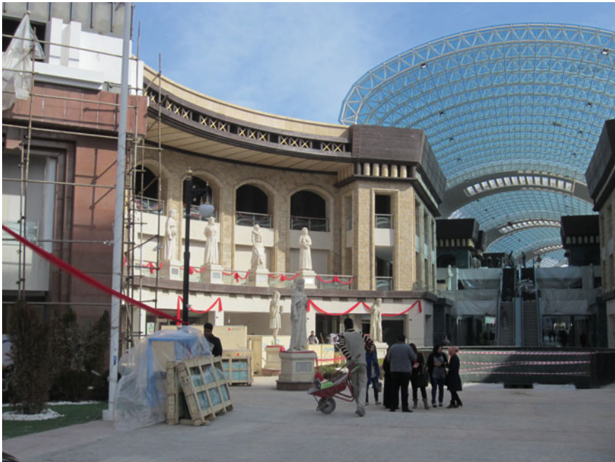
Fig. 6.3 Finishing works in the Plaza fronting the new Erbil Downtown development
