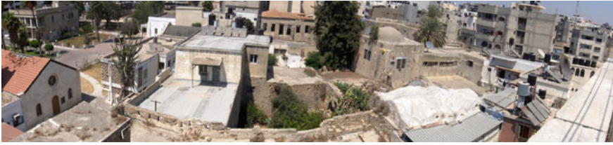
Fig. 10.2 The compact fabric of houses in the Old City. Source Authors
