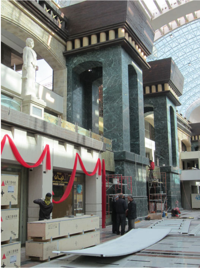
Fig. 6.4 Interior of the new Erbil Downtown development
