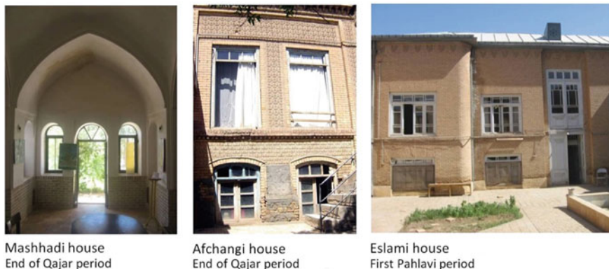
Fig. 11.4 Changes in the size, proportions and positions of windows under the influence of European architecture compromised the thermal performance of the buildings. Source of photos Estaji (2017)
