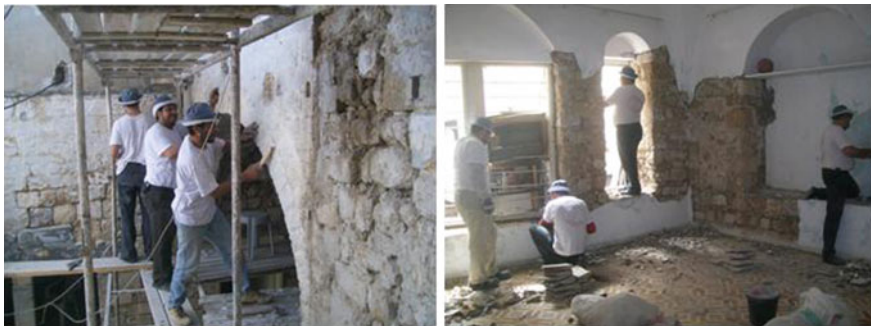
Fig. 14 Removing the cement layers
