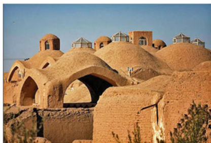
(b) House in Zavvare: semi-open central space
