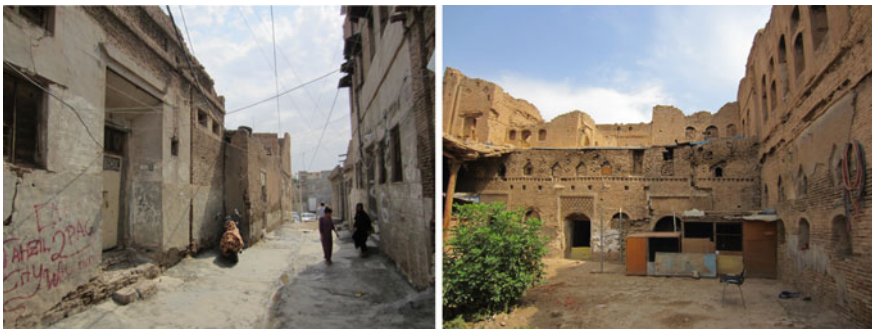
Fig. 6.1 Without its inhabitants the overall building stock and the existing infrastructure are rapidly deteriorating
