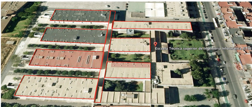
Fig. 2. School of Computer Engineering building
