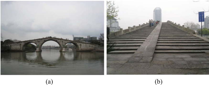
Fig. 26.1 The Gongchen Bridge. (a) Side view. (b) Front view
