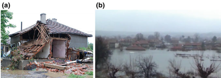
Fig. 13.11 Floods resulting of artificial structures damages: a Tzar Kalojan village, Aug 2007, b Biser village, Feb 2012; (Chilikova-Lubomirova et al. 2017)
