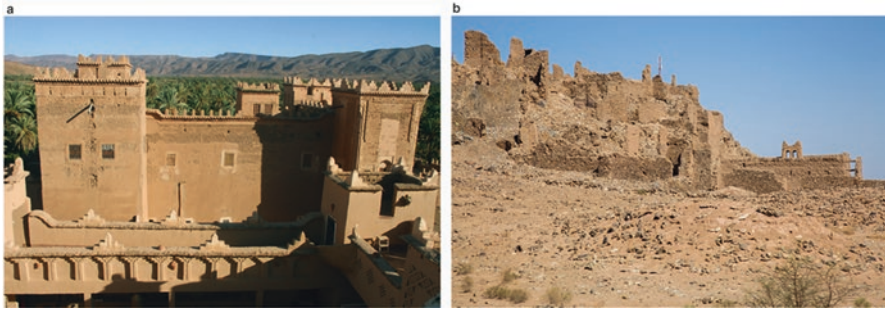
Fig. 15.3 (a) Restored Kasbah in Agdz; (b) Decayed earthen buildings in rural areas (Photo credits: M. Maurissens)
