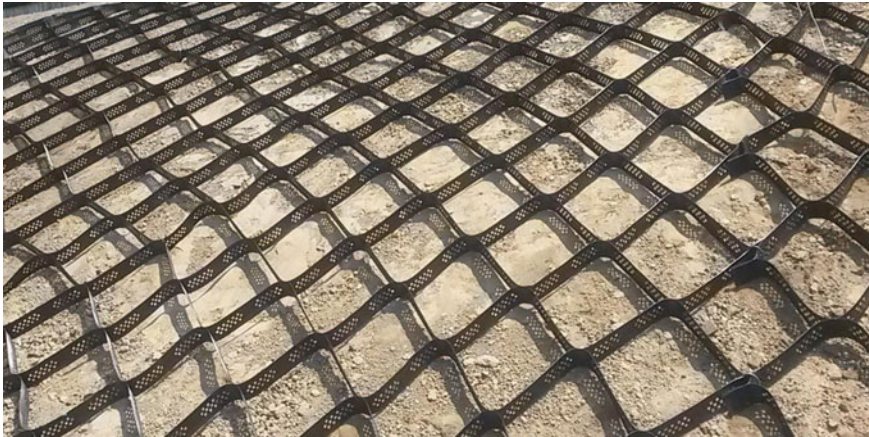
Fig. 13.15 Anti-erosion network of synthetic material
