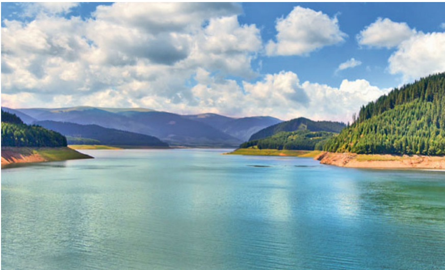
Fig. 15.6 Vidra Reservoir, which supplies the Ciunget Hydropower Plant on the Lotru River
