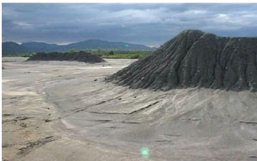
Fig. 3.34 The central part of Aurul Tailing pond (2014) [17]
