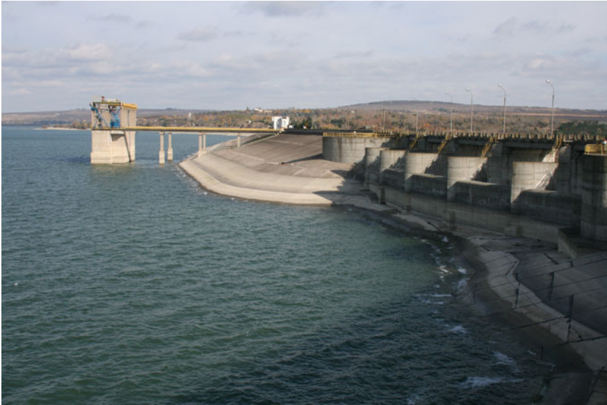
Fig. 15.3 The dam at Stanca-Costesti on the Prut river
