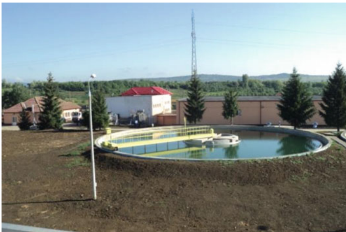
Fig. 6.7 The modernized Vârșolț WTP (photo by courtesy of CAS S.A.)
