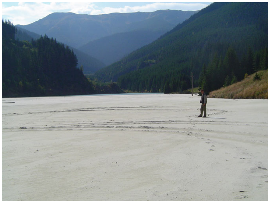
Fig. 3.31 The Dumitreleu sediment retention reservoir (2008)
