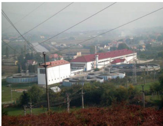
Fig. 6.12 The Gilău WTP (photo by courtesy of CAS S.A.)
