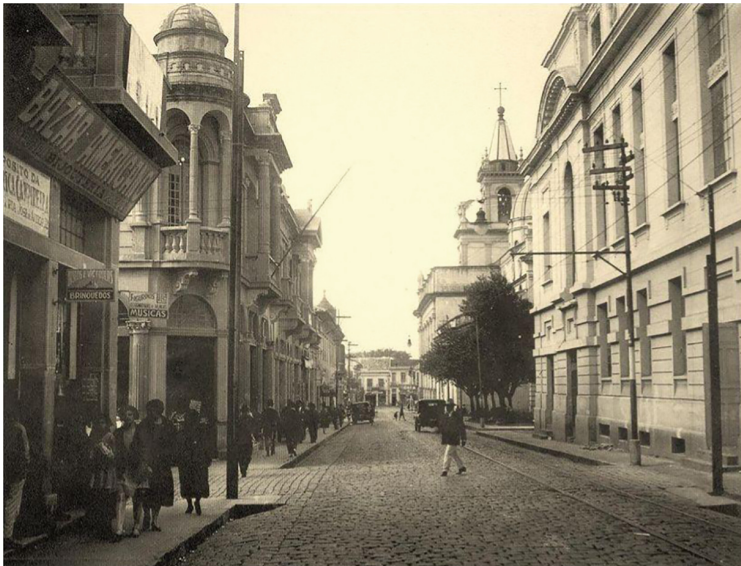
Fig. 4. Treze de Maio Street, in which the Salles Pharmacy is located, on the block to the side of the Cathedral. Source: CCLA archive.
