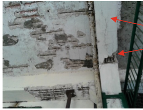
Photo 4 Loss of the clear cover reinforcement in concrete slabs and beams, corrosion of the reinforcement steel, cracking of the concrete and large deformations in the reinforced concrete elements
