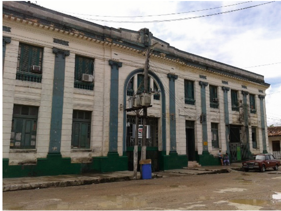
Photo 1 Facade of the reparations building, TRANSCUPET, Caibarién (built in 1922)
