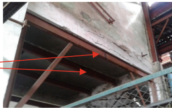
Photo 5 Reinforced concrete beam with loss of the clear cover reinforcement steel, corrosion of the reinforcement steel, cracking of the concrete and large deformations, element with structural failure
