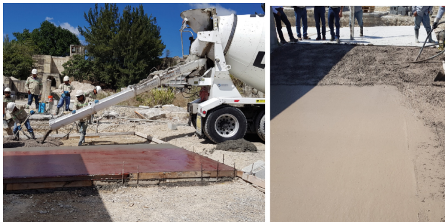
Fig. 8 Application of the ready mix of LC3 concrete
