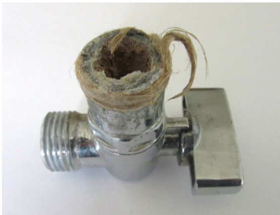
Fig. 35.1 Corrosion area on a section of a fitting with precipitate on the surface
