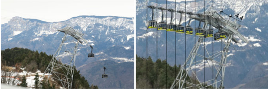
Fig. 1 Left: Areal cable ropeway with two vehicles passing over the same support at different times and different driving directions. Right: a picture sequence to visualize the oscillations when the vehicle passes the support (photo Doppelmayr )
