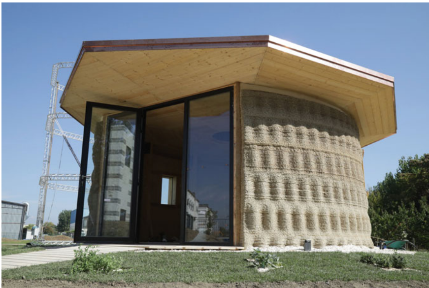
Fig. 8 3D printed the Gaia House [33]
