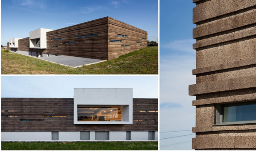
Fig. 6 Use of cork for external cladding. Logowines Winery (Evora, Portugal, 2009, PMC Arquitectos) [26]
