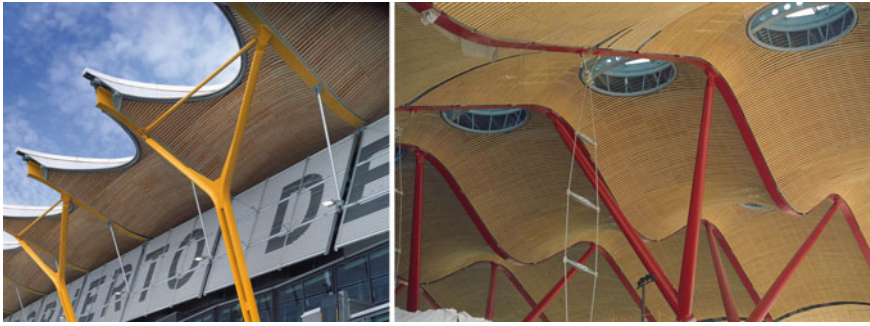
Fig. 4 Use of engineered bamboo for cladding in the Terminal T4 of Madrid Barajas Airport [11]
