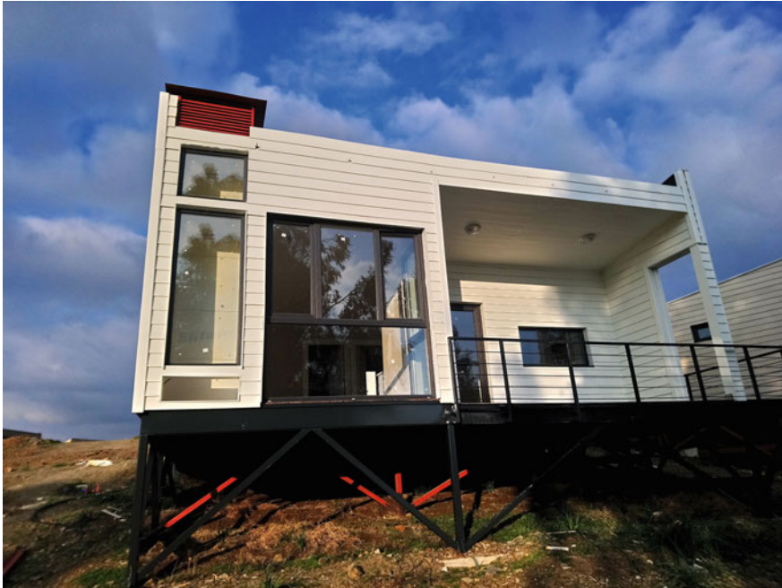
Fig. 4 The solar chimney system placed on the South facade (the left side of the picture)
