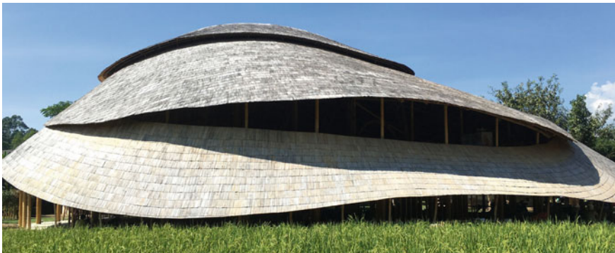
Fig. 10 Bamboo Sports Hall of Panyaden International School [35]
