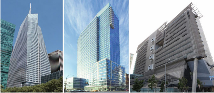
Fig. 5 LEED-certified green buildings that include the partial replacement of cement with SCM. a The Bank of America Tower—45% blast-furnace slag, b The Helena—45% blast-furnace slag, c San Francisco Federal Building—50% blast-furnace slag
