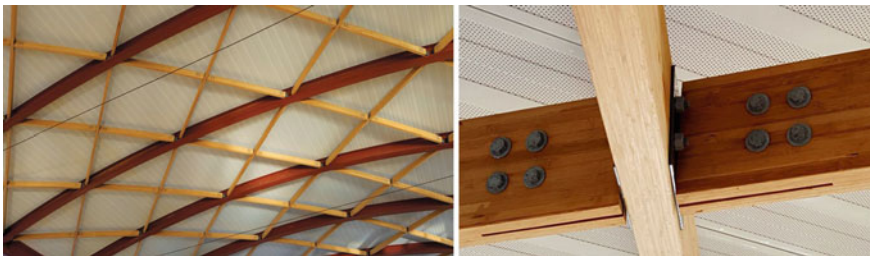
Fig. 3 Use of engineered bamboo for the structural system in the Terminal of the Veterans Airport of Southern Illinois [9]
