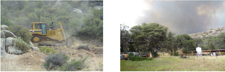
Fig. 4. a & b (left) June 30, 2013, 1348 h., Yavapai County Morin dozer building fireline in The Shrine area. Source: Anonymous By Request FF. (right) June 30, 2013, 1437 h. Peeples Valley FD Water Tender and unknown Municipal FD Type 6 Engine in The Shrine area. The BRHS are to the left in the trees out of view. Source: Anonymous By Request FF.
