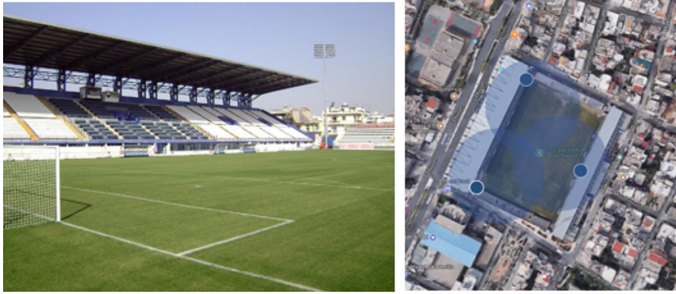
Fig. 4. (left) Egaleo municipal stadium; (right) Placement and coverage of radio cells
