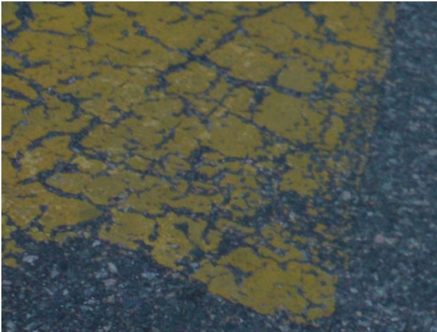
Fig. 1.5 Painted street line
