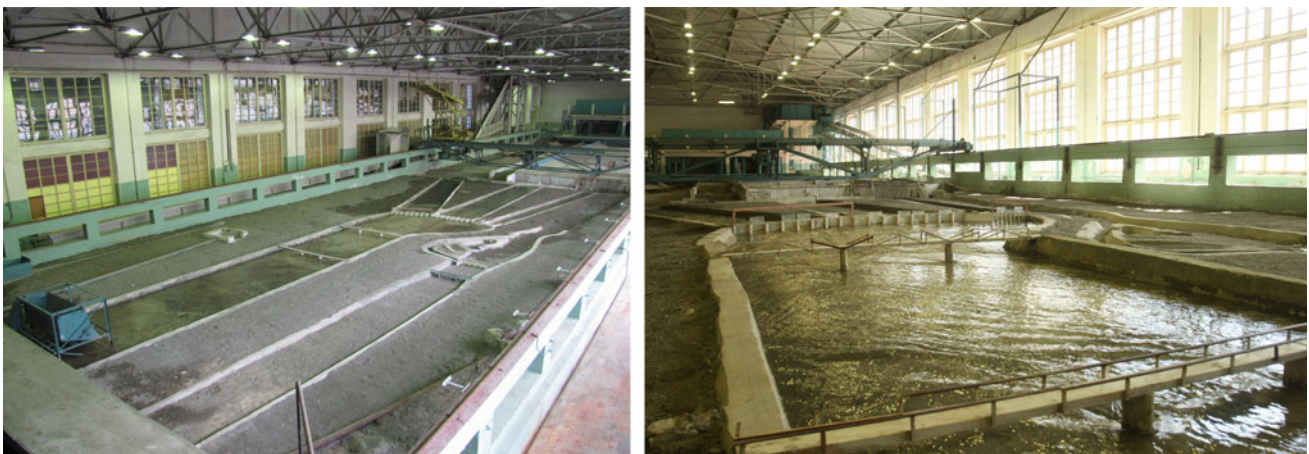
Fig. 2.11 Laboratory of Hydraulic Engineering of the Water Management Institute. Photo by G. Gavardashvili
