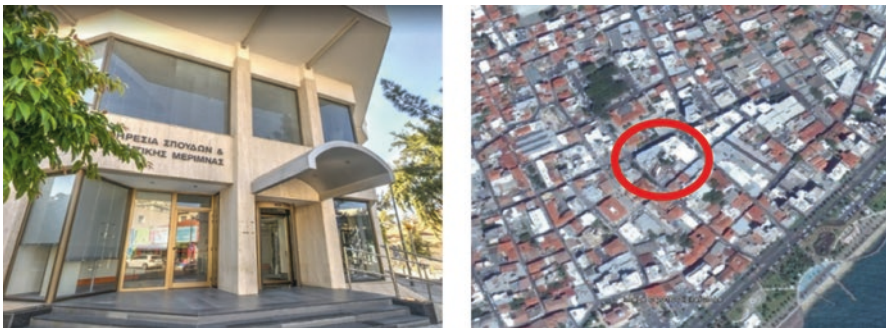
Fig. 5.1 (1) Limassol building (left); (2) Limassol urban isle area (inside red circle) (right)
