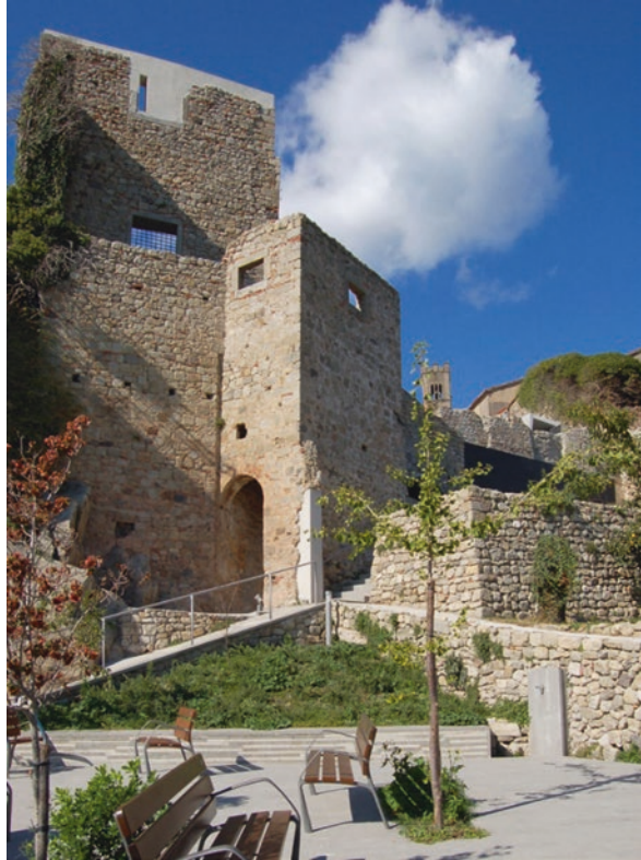
Fig. 37.7 Santa Fiora Village in Tuscany. View of rehabilitation actions of courtyards, towers, walls and house buildings, according to the valorization of environmental performance
