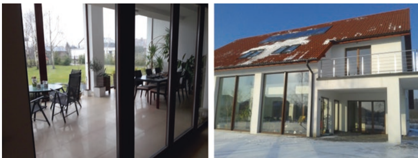
Fig. 80.2 Solar buffer space incorporated into the interior of a building, view from inside (in summer) and from outside (in winter)
