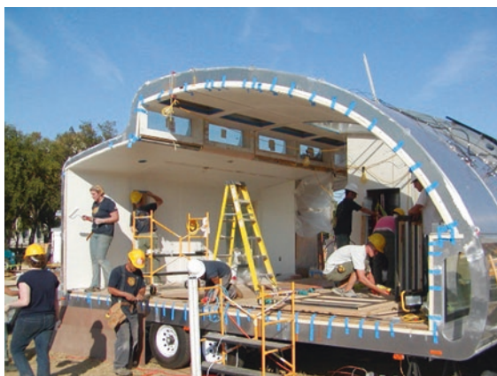
Fig. 14.8 The Michigan Solar House (MiSo) during its construction (D. Oktay Archive)
