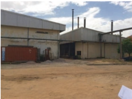
Plate 20.1 A gable roof, monitor roof and shed roof at Funtua textile limited (Source: Author's field work)
