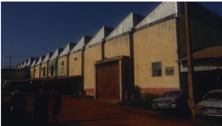
Plate 20.9 Factory building with rectangular plan and saw-toothed roof (Source: Author's field work)
