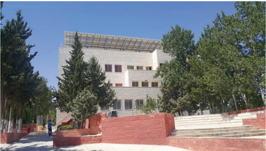
Fig. 52.6 A good example of the photovoltaic panels placed on the roof of a building at Al-Ahliyya Amman University; it was accepted by people (source: research)
