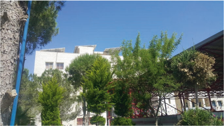
Fig. 52.12 A bad example of the photovoltaic panels placed on the roof of a building at Al-Ahliyya Amman University and affected the elevation; it was rejected by people (source: research)
