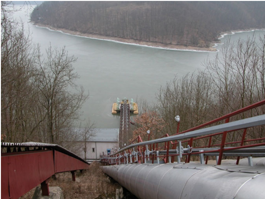
Fig. 7.5 Floating ponton in Vranov reservoir
