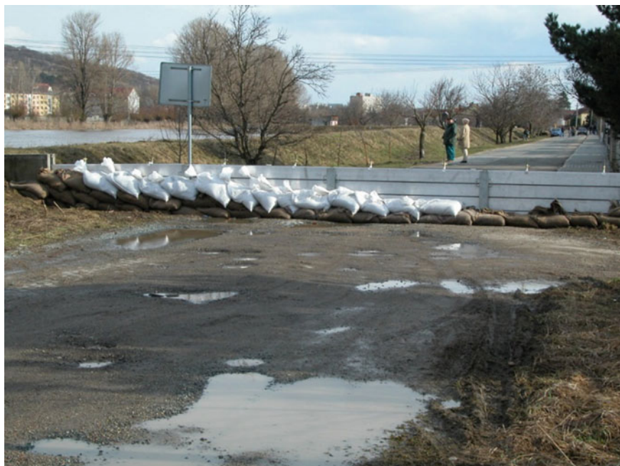
Fig. 7.13 Spring area Vojkovice—flood protection
