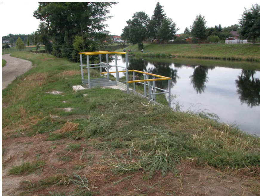
Fig. 7.12 Water intake from the Jihlava River
