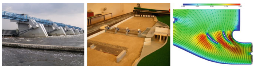
Fig. 2.13 Weir and the small hydroelectric power plant Štětí (a prototype, a physical model and a numerical model)
