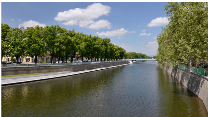
Fig. 14.5 The regulated Labe in the city of Hradec Králové—as an example of subjective perception and the paradox of ecosystem disservices. The river binding between firm walls is part of flood protection and the reinforced silting permits recreational enjoyment close to the water surface. On the other hand, the straightened and monotonous river basin is aesthetically dull and makes the Labe a canal more than a river. Ecosystem disservice (the non-aesthetic nature) of the watercourse is, therefore, a consequence of anthropological activity—river basin adaptation—done to suppress another ecosystem disservice (erosion and floods). Photograph: Jiří Schneider
