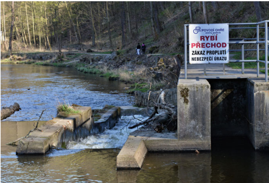
Fig. 15.5 Maintaining migration corridor on the river Ohře—under Ohře River Board, s. e. administration. (Photograph: Jiří Schneider)
