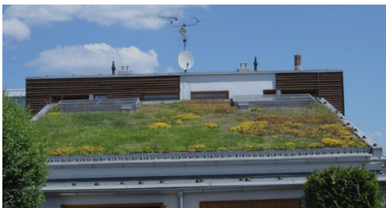
Fig. 3.3 Roof with extensive planting (Source Kotásková)
