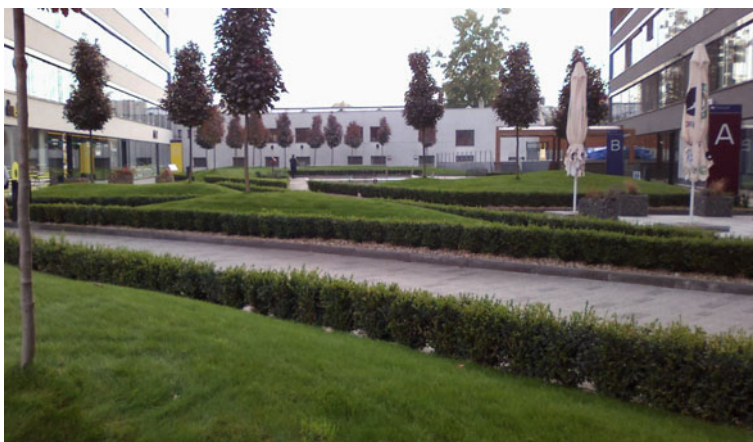
Fig. 3.2 Roof with intensive planting (Source Kotásková)
