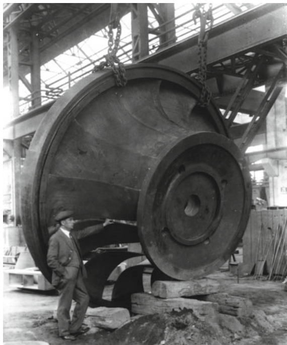
Fig. 15.16 Historical photograph of a Francis turbine runner for a SHPP Mířejovice
