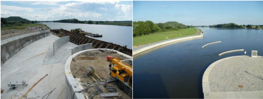
Fig. 15.8 Intake part of the SHPP Litoměřice under construction (left) and after completion (right)
