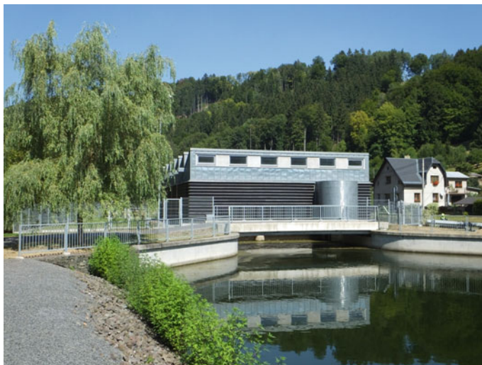
Fig. 15.30 Powerhouse of the SHPP Železný Brod from the intake side
