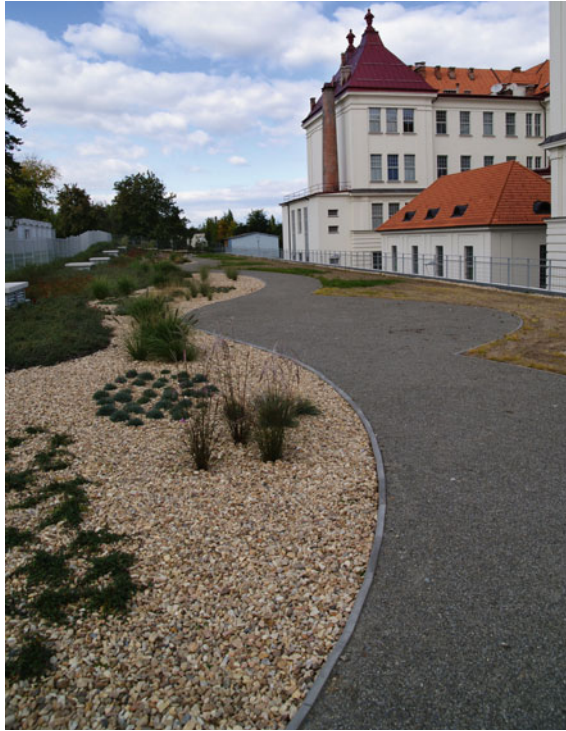
Fig. 4.1 Surface infiltration—Brno University of Technology Campus, CR
