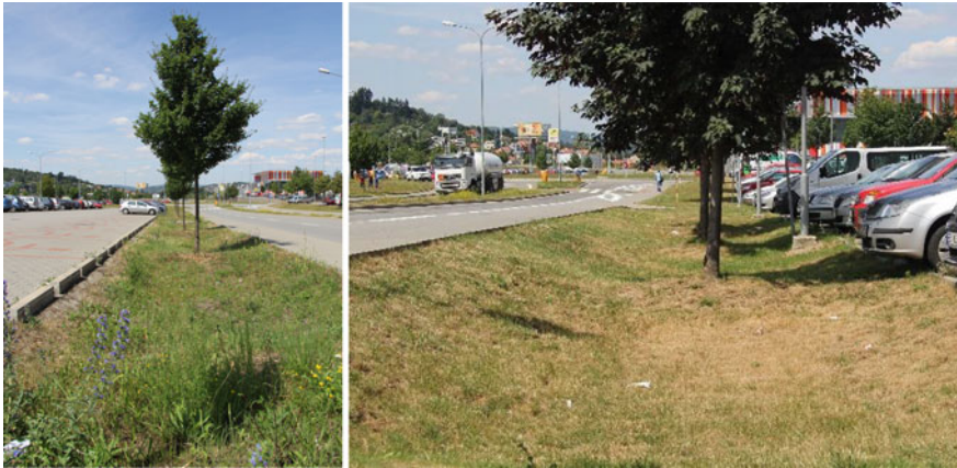
Fig. 4.5 Trench (furrow) infiltration—Campus, Brno, CR
