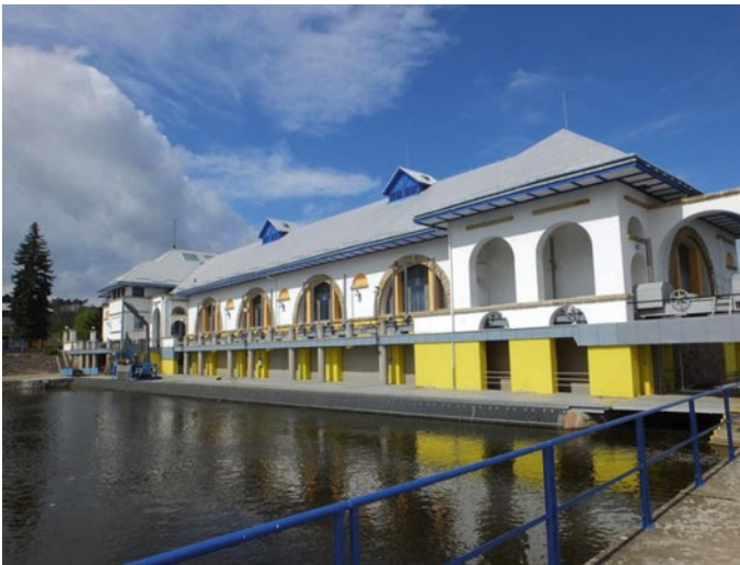
Fig. 15.10 Powerhouse of the SHPP Měřejovice from the intake side
