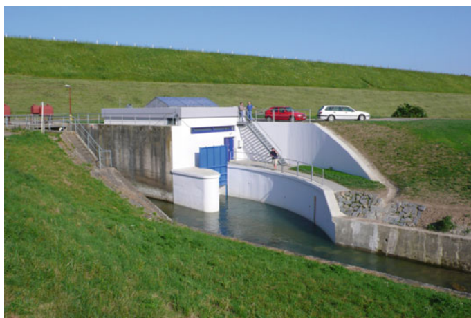
Fig. 15.19 Powerhouse of the SHPP Rozkoš from the outlet side (source Hydrohrom, s.r.o.)
