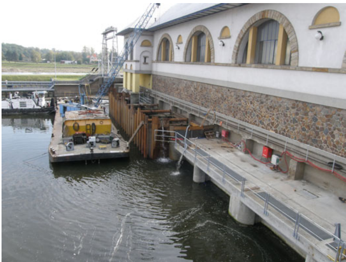
Fig. 15.18 Construction works on the outlet part of the SHPP including modification of the draft tubes of turbines and installing new draft tube stop logs
