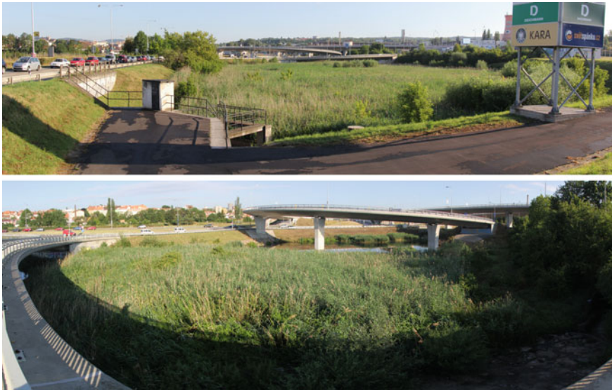
Fig. 4.7 Infiltration basin with a reservoir for sedimentation—Královo pole, Brno, CR
