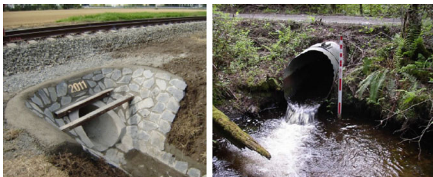
Fig. 11.14 Culverts (a typical and non-environmental solution) [35]
