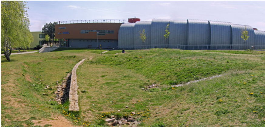
Fig. 4.3 Swale infiltration—Kohoutovice, Brno, CR
