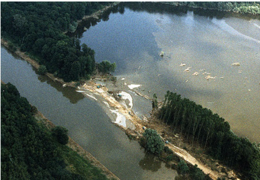
Fig. 14.1 Collapsed levee close to Kvasice on the Morava River
