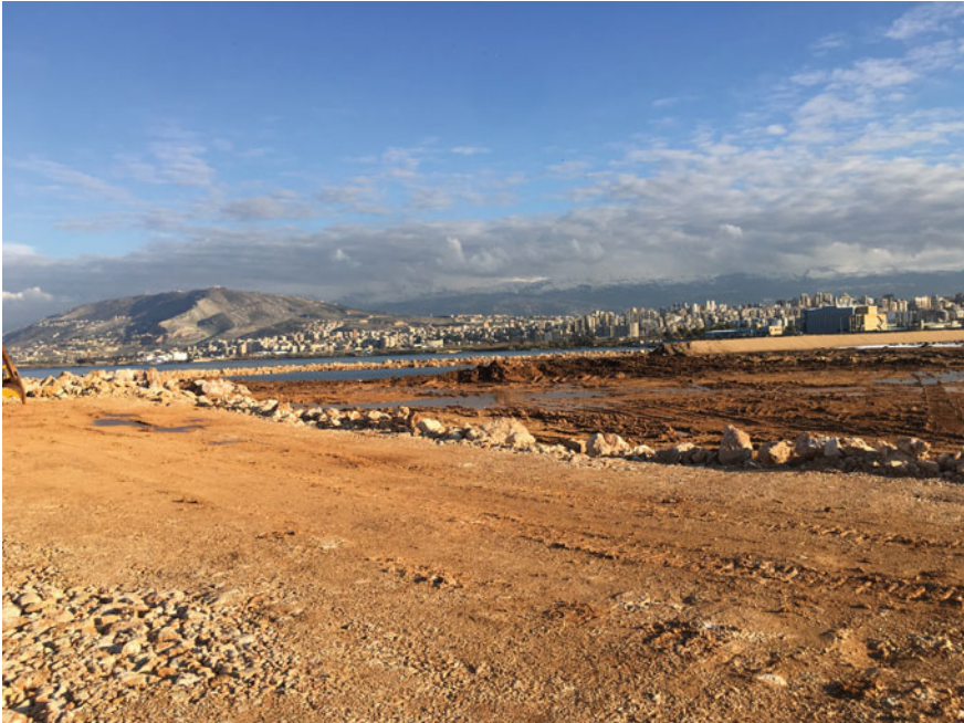
Fig. 11.12 Reclaim to build a new temporary sanitary landfill in Tripoli
