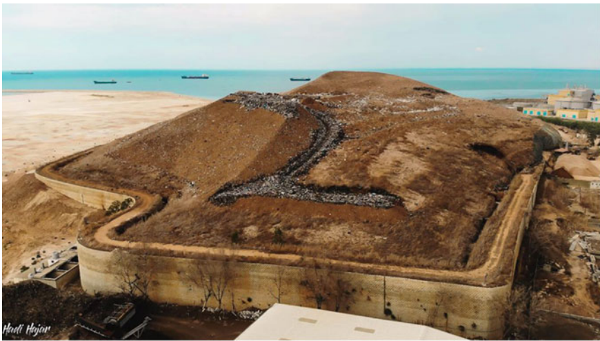
Fig. 11.3 Aerial view of Tripoli Landfill
