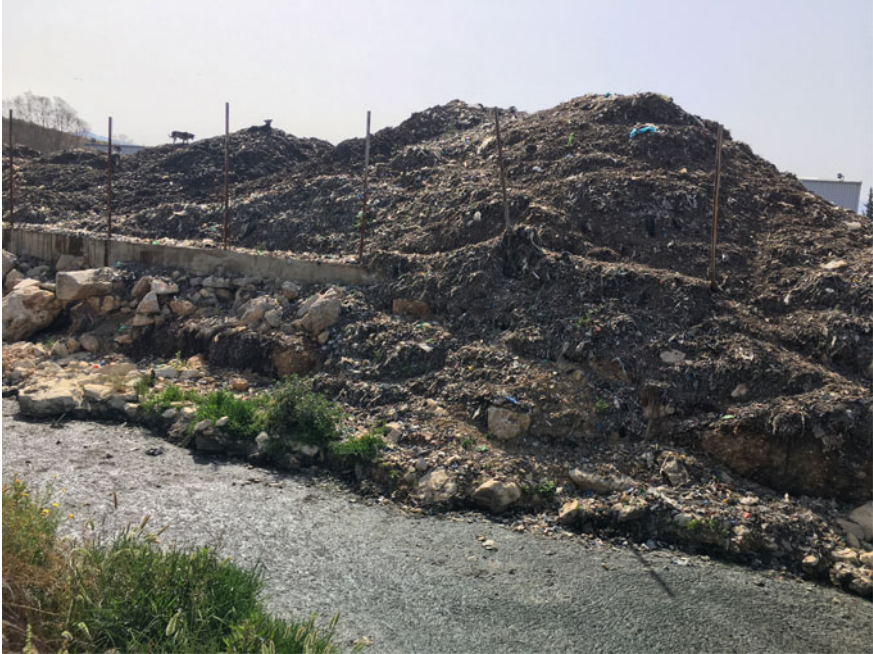
Fig. 11.10 None conform compost produced in Tripoli composting facility with leachate in open air
