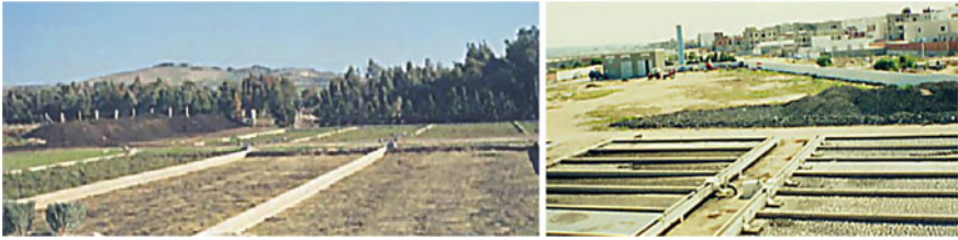
Fig. 3.4 On-site disposal/storage of biosolids in the treatment plants. Courtesy of Olfa Mahjoub (2013)
