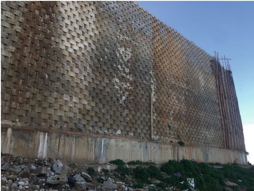
Fig. 11.7 Part of the peripheral wall in Tripoli Landfill
