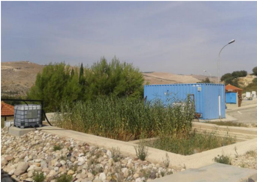
Fig. 15.8 Plant acclimatization phase in sludge drying beds during operation at Fuheis Facility site
