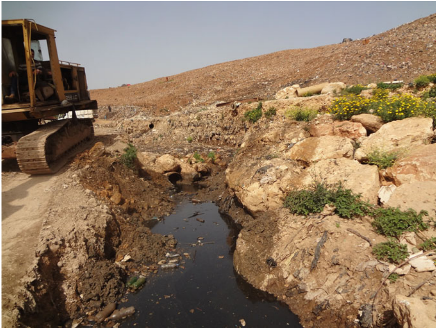
Fig. 11.5 Leachate discharged to the Abou Ali River
