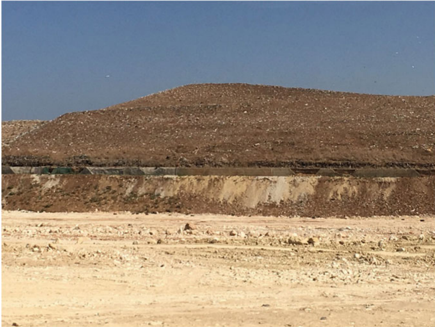
Fig. 11.9 Additional protection built in front of the collapsed peripheral wall
