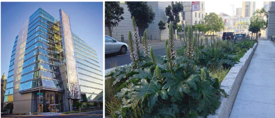
Fig. 4.3 SFPUC building and outdoor constructed wetlands for onsite treatment
