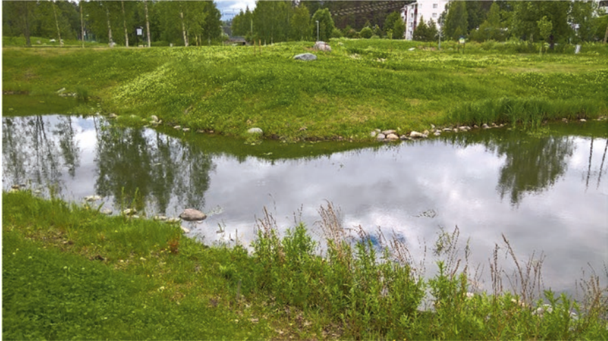
Fig. 2.9 The Eerolanpuro engineered wetland in Jyväskylä, Finland, attenuates pollutants in stormwater runoff before discharge to nearby Lake Tuomiojärvi, which serves as a source of raw water for the city
