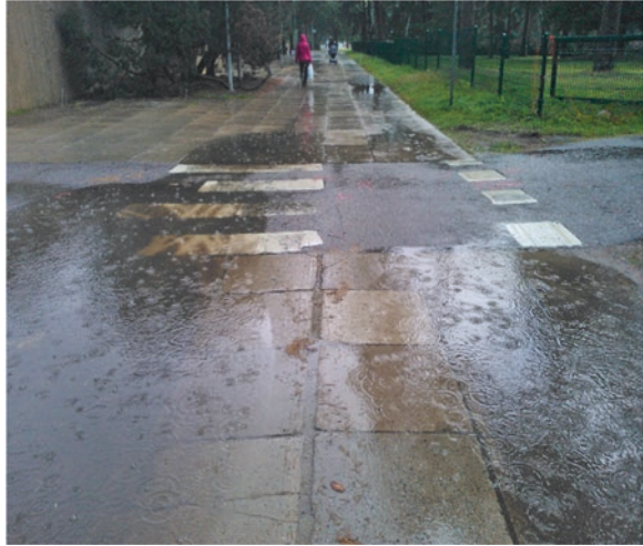
Fig. 2.1 Surface sealing in urban areas reduces infiltration (near field), increasing stormwater runoff and flood risk
