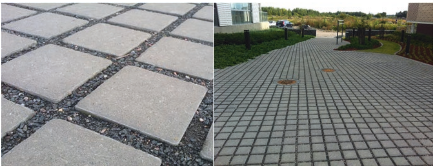
Fig. 2.5 Water infiltrates permeable interlocking concrete pavement through openings between pavers
