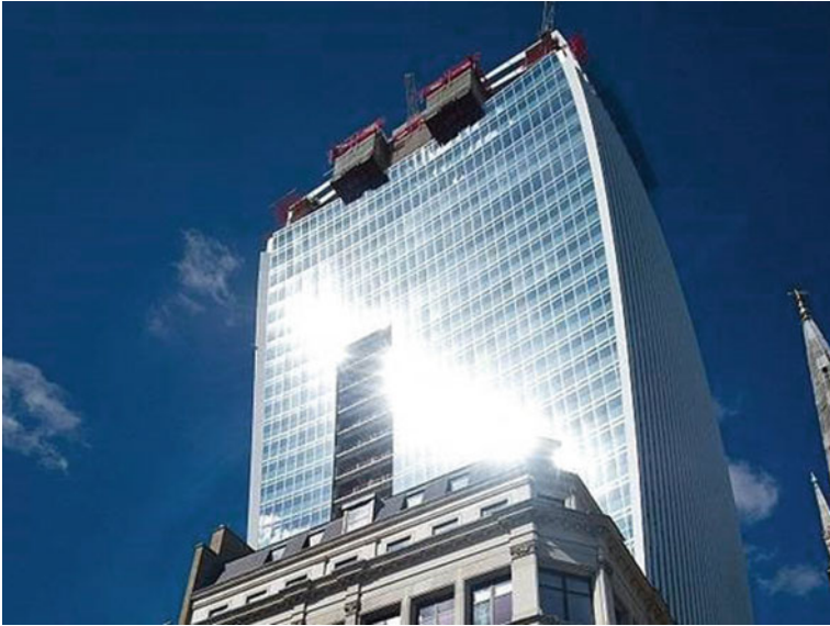
Fig. 6.16 London's 20 Fenchurch Street tower. Source Nvidia
