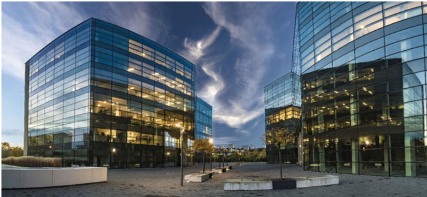
Fig. 6.29 Modern office buildings. Source Mike Mareen
