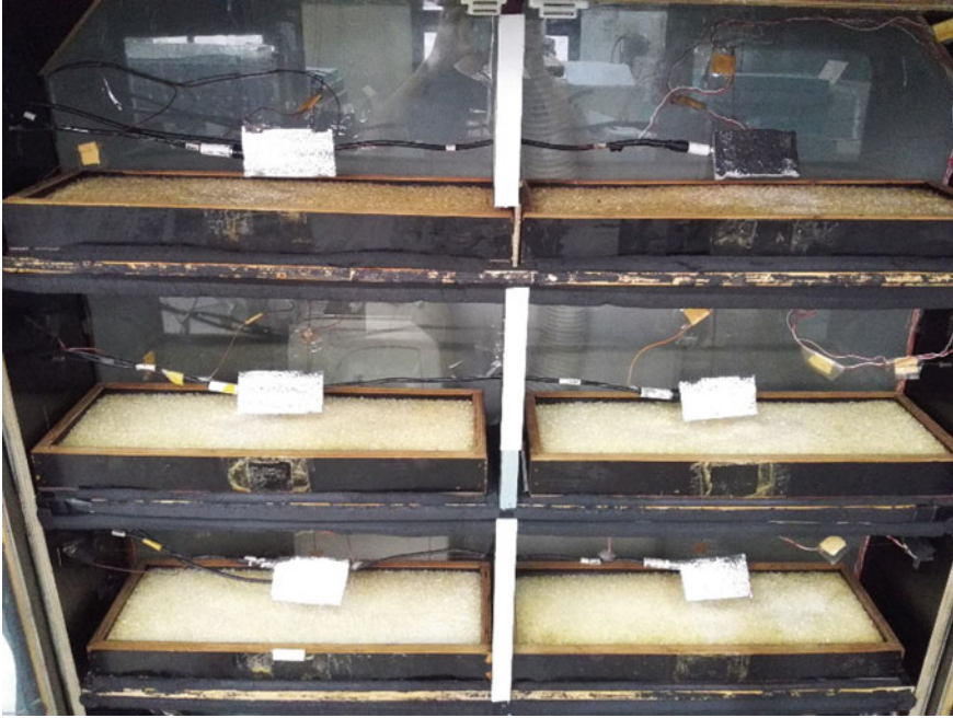
Fig. 44 Image of the desiccant modules embedded in the window
