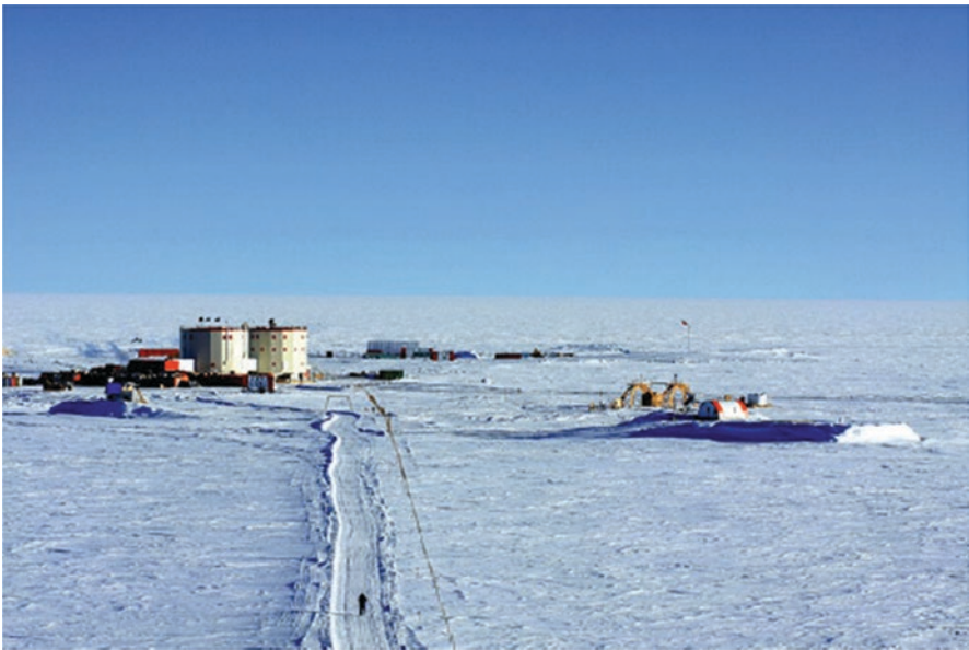
Fig. 38.1 Concordia station. The two principal towers can be seen; the “noisy” tower which houses life support, recreation, food storage and preparation, and the mess; the “quiet” tower which houses sleeping quarters, laboratories, and medical
