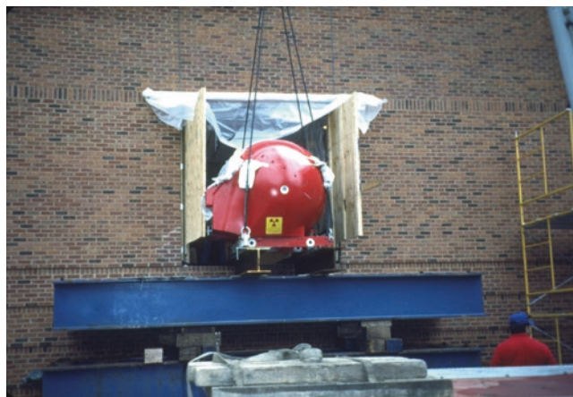
Fig. 1 Gamma Knife® Model U (Elekta, Stockholm, Sweden) at the University of Virginia being prepared for source reloading. The clamshell design of the unit required it be removed from the treatment vault and placed in a temporary bunker
