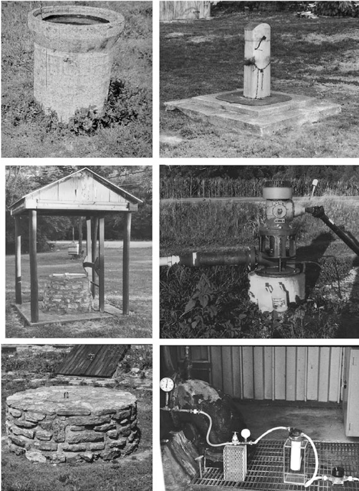
Fig. 8.3 This figure shows wells that provide water for groups with different levels of need and the wells show different levels of sanitary protection. Upper left is an artesian flow well in the Cauca River valley region of Colombia. Center left is a covered bucket well under a roof shelter near Oxford, Ohio, USA. Lower left is a capped bucket well near Cincinnati, Ohio, USA. Upper right is a sealed well with a hand powered pump near Cincinnati, Ohio, USA. Center right is a sealed well operated by the drive shaft of a farming tractor in Hamilton county, Ohio, USA. Lower right is a sealed well within an enclosure in Butler County, Ohio, USA, and this view shows that water in the well head was being sampled for possible viral contaminants. Use of these images is courtesy of the author
