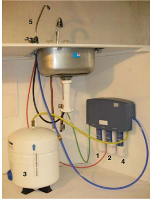
Fig. 8.34 This image is titled “A typical home RO system” including (1) particle filter, (2) reverse osmosis membrane unit, (3) pressurized treated-water storage container, (4) carbon adsorption post-filter and (5) separate treated-water tap. It is by North Dakota State University, authors Roxanne Johnson and Tom Scherer, and being used under a Creative Commons Attribution-share alike 3.0 license. https://www.ag.ndsu.edu/pubs/h2oqual/watsys/wq1047.pdf
