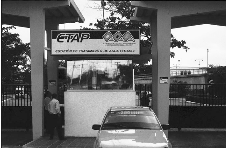
Fig. 8.16 This image shows the entrance to the Barranquilla, Colombia rapid sand filtration drinking water treatment plant. Use of this image is courtesy of the author
