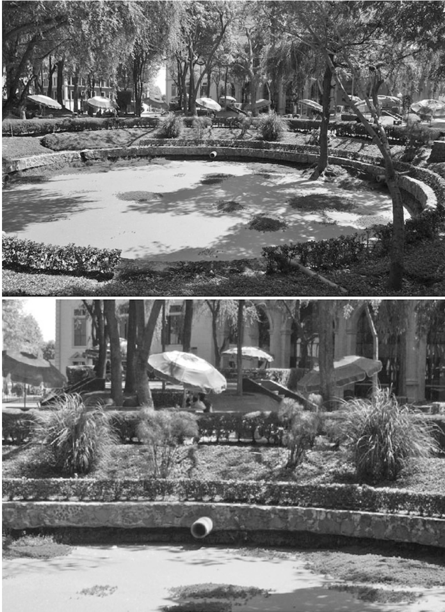
Fig. 8.9 This figure shows the receiving basin for a rainwater ground catchment system. The lower image is a magnification of the upper image, and better shows the water inlet pipe. This image is titled “03242012Taller sostenibilidad lore037” by Talento Tec and used under the Creative Commons Attribution 3.0 Generic license. The text described this as being a cenote, which suggests that it may be an adapted sink hole
