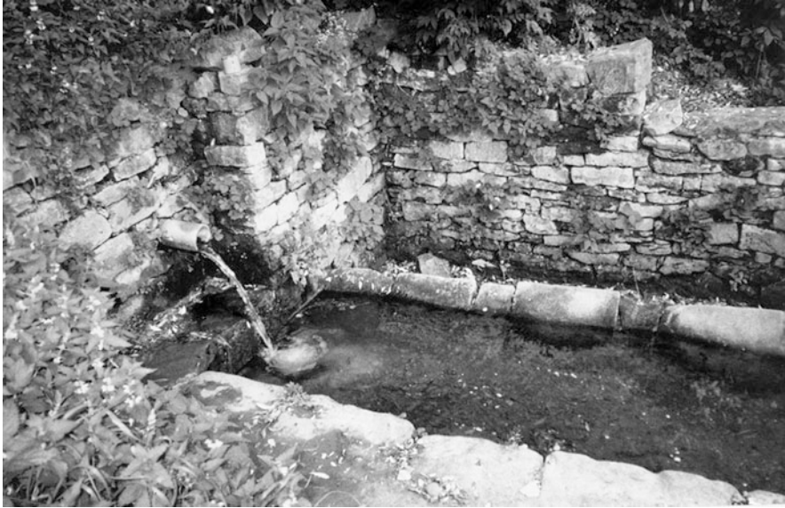
Fig. 8.7 This image shows water from a spring which is being conducted by means of a horizontal well pipe into a collection pool. This spring is the water source for the village Dzyhivka in Ukraine. The image is titled “Siphot” by USchick and being used under a Creative Commons Attribution-share alike unported license. 3.0 Generic license
