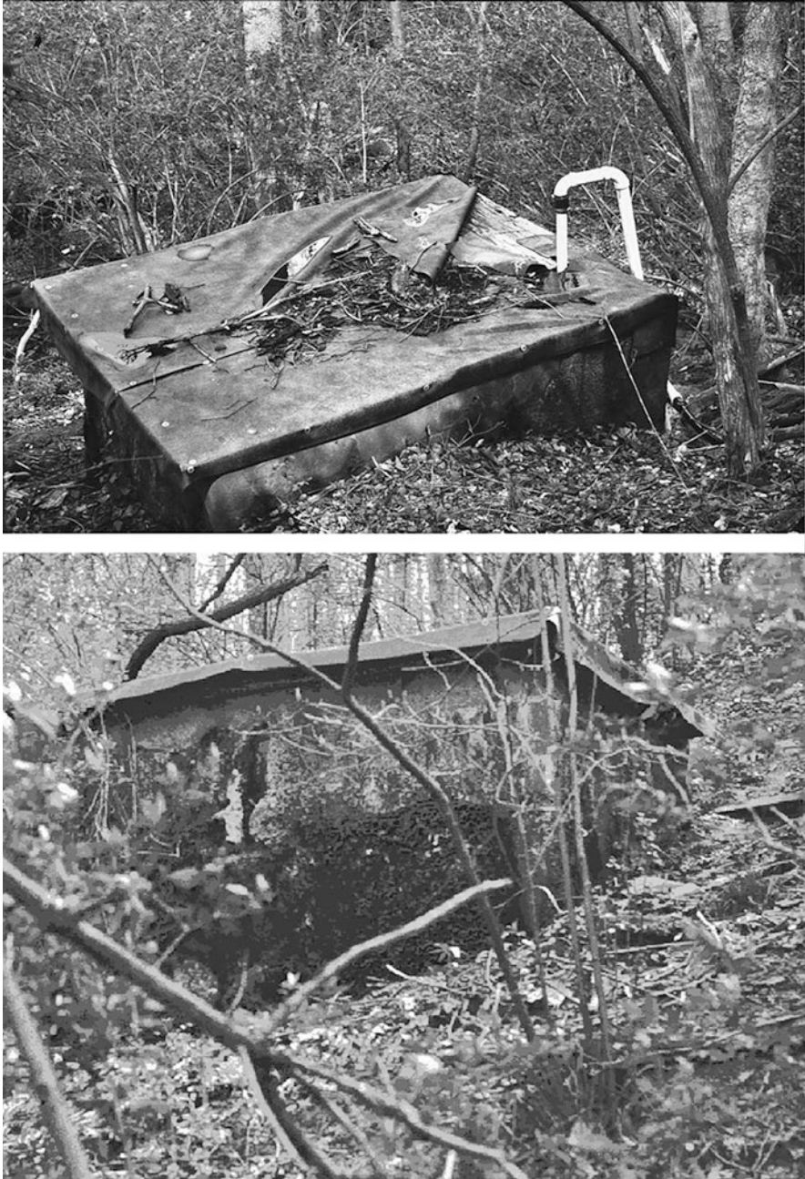
Fig. 8.6 These images show a spring water cistern, sometimes called a “Spring box”, which intercepts and stores for distribution the water that emerges from a hillside spring near Cincinnati, Ohio. Use of these images is courtesy of the author
