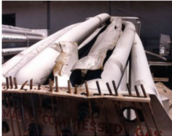
Fig. 6.1 Close up view of tube bank, post-accident [4]
