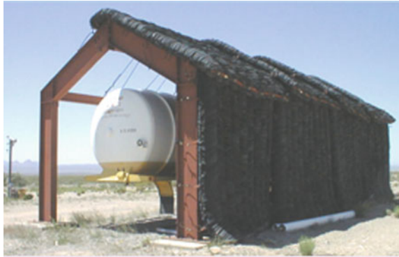
Fig. 6.20 Blast mat used to protect a LH 2 trailer from shock and shrapnel [4]
