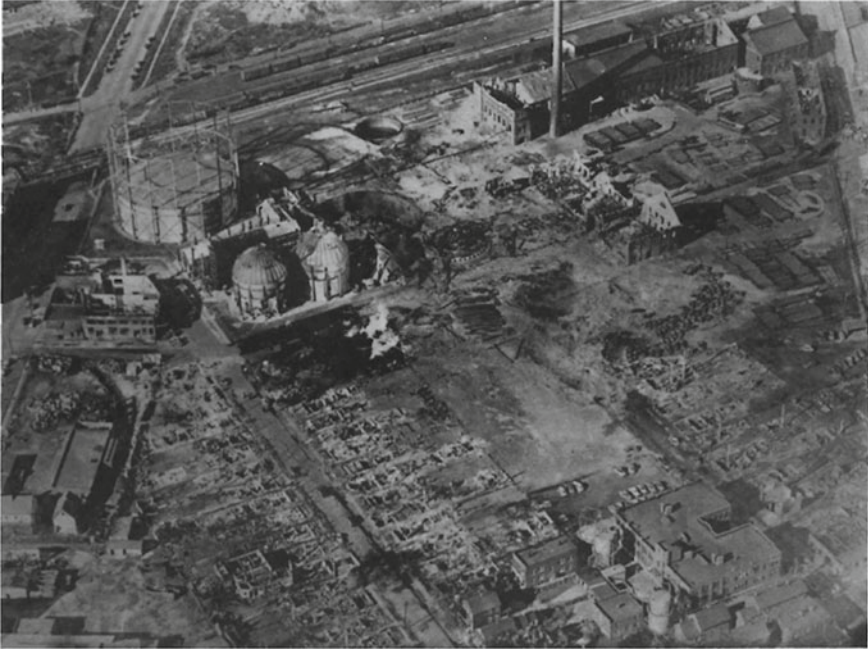
Fig. 1.1 Resulting damage from the 1944 Cleveland LNG Fire and explosion. Gas plant located in the upper half of the picture; note destroyed homes, factories and other buildings in the lower half [2]
