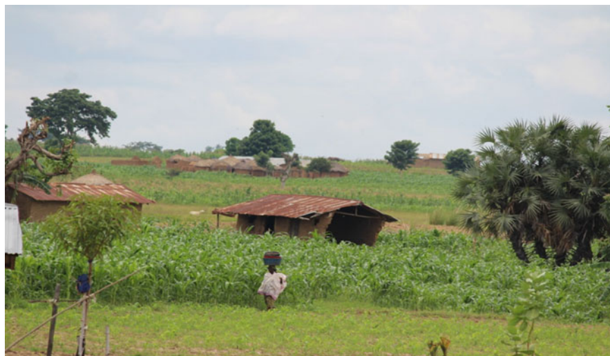
Plate 3 Another Image showing affected houses and farmlands by the flood. Source: field survey, 2013
