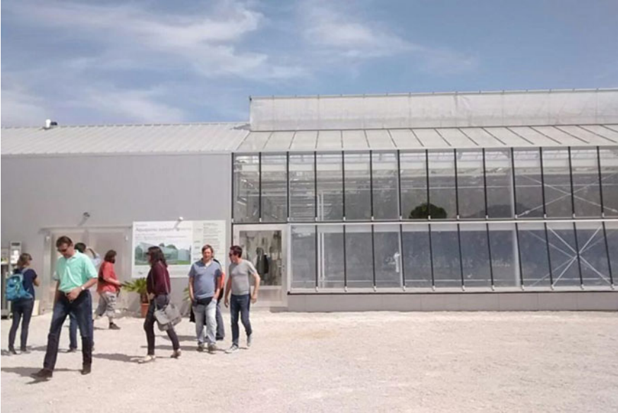
Fig. 21.10 INAPRO aquaponics enclosure with two sections, opaque for fish and greenhouse for plants (Murcia, Spain)
