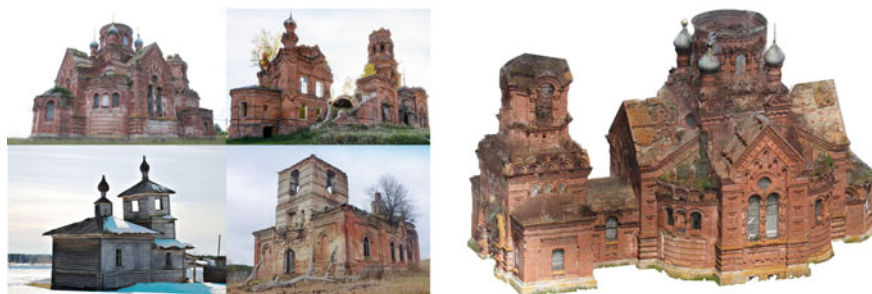
Fig. 7 Some examples of religious architecture dispersed in the Upper Kama Region and 3D model of the Taman church obtained with SfM detection
