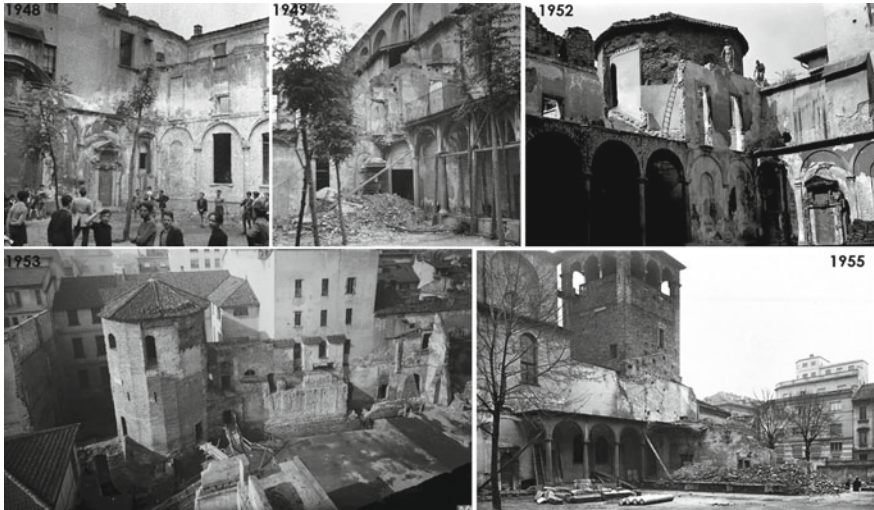
Fig. 3 The transformations of cloister of the Monastery of St. Maurizio in the years following the Second World War
