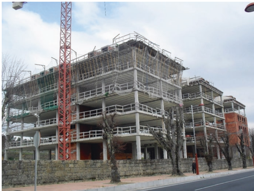
Fig. 8.4 One of many abandoned construction sites, in O Carballiño, Galicia, Spain, in 2013. (Photo: João Queirós)
