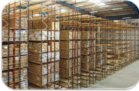
Fig. 4.5 Adjustable pallet racking
