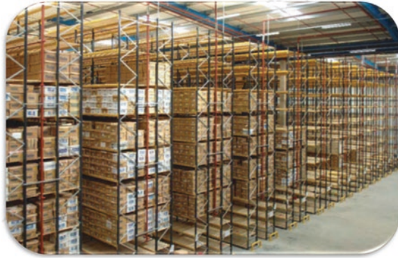
Fig. 4.5 Adjustable pallet racking
