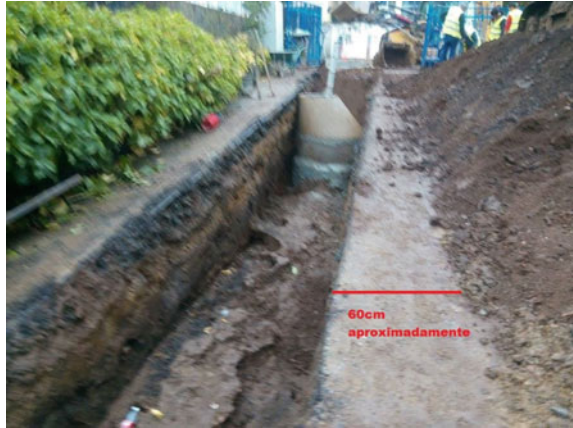
Fig. 3 Safety distance to the trench
