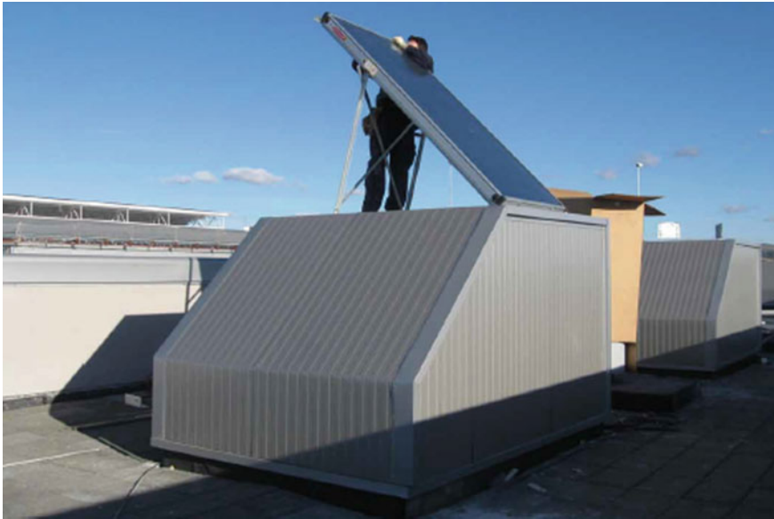
Fig. 1 Installation of the glass cover
