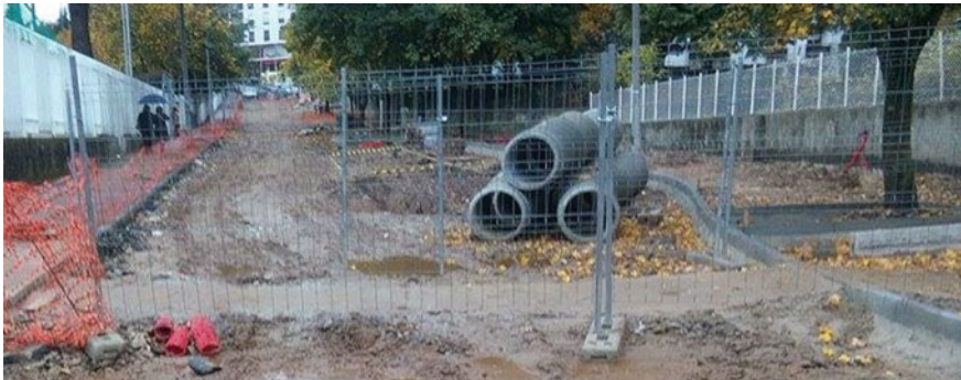
Fig. 4 Fencing of the work
