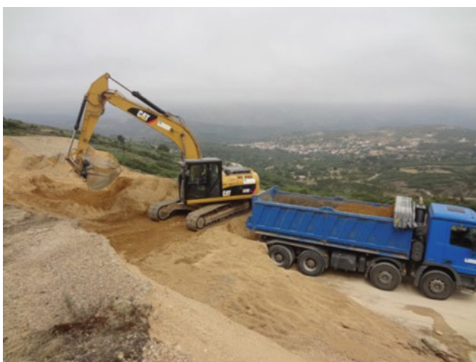
Fig. 2 Removal and transport of uranium milling waste from the old mine and milling site of Forte Velho, Guarda
