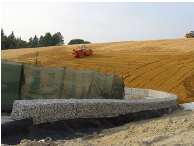
Fig. 1 Recontouring the uranium milling waste pile of Urgeiriça (Barragem Velha) and compacting the soil layers of the cover
