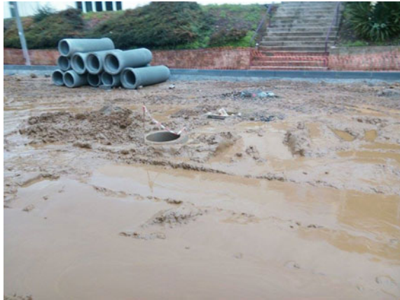
Fig. 2 Placement of a shackle to aid in the flow of water
