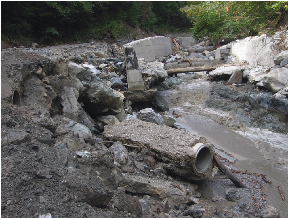
Fig. 17.11 Impact of a torrential flood in the Davča Valley (Škofja Loka Hills) in 2007. (Photo by Matija Zorn, GIAM ZRC SAZU Archive)
