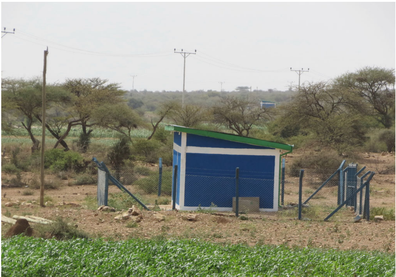
Fig. 7 Battery of the wells newly drilled for the city of Jijiga
