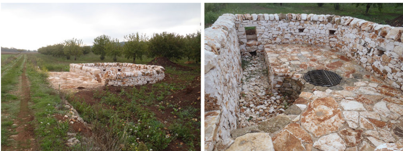
Fig. 3 The access to the cave, after the works to ensure safe entrance to the system
