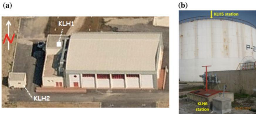
**Fig. 13.26** **a** The municipal gymnasium building (Bing Maps Image) and **b** the steel water tank located in the broader urban area of Kalochori, west of Thessaloniki. The locations of the accelerometric stations are also shown
