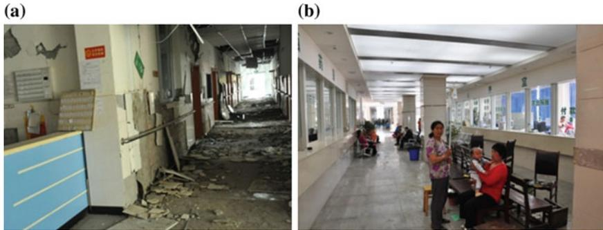
**Fig. 5.2** The Lushan county hospital (China) **a** damage suffered by the conventionally founded buildings; **b** full integrity and operability of seismic isolated building
