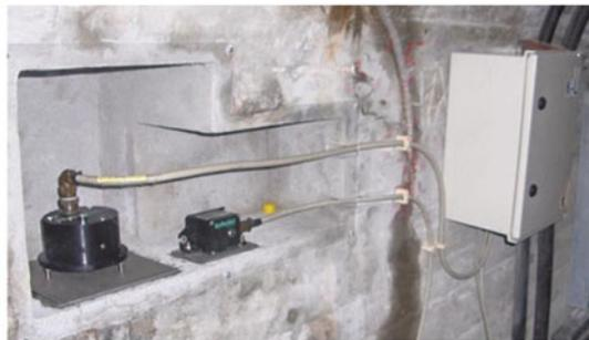
**Fig. 4.11** Cabril dam. Vibrations monitoring system—schematic representation and main hardware components
