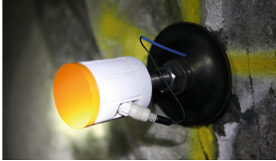
Fig. 1 IoT-enabled rock bolt installed in mine tunnel
