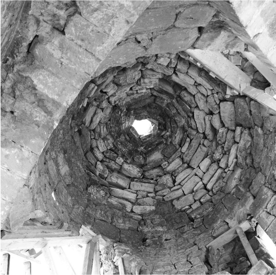
Fig. 1. Hagia Marina dome (before restoration) in Nicosia, Cyprus.
