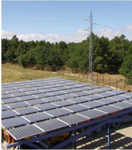
Fig. 2. Photovoltaic system integrated in the rooftop of the parking area of CEDER in Lubia (Soria, Spain). Image courtesy of: CEDER.
