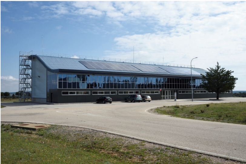
Fig. 1. Photovoltaic system in the rooftop of the offices of CEDER in Lubia (Soria, Spain). Image courtesy of: CEDER.
