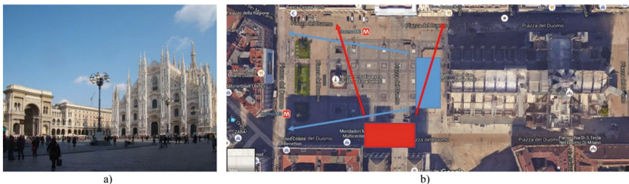
Fig. 39.1 The square of Duomo (a) and the layout of the stages (b) for the concert season (Pop/Rock concert in red, symphonic music in blue) with sound propagation directions
