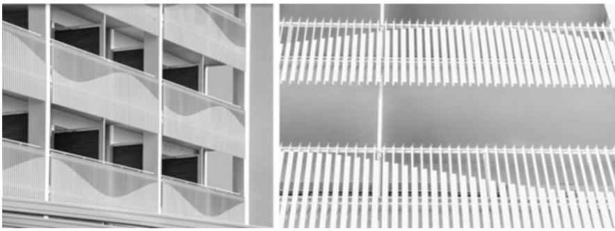
Fig. 3 Balcony rail/sunshade system, “Archigraph” design (Photography source F. Psychopoulou)
