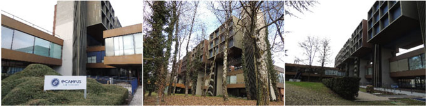
Fig. 1. The building complex of University eCampus (architect Bruno Morassutti)
