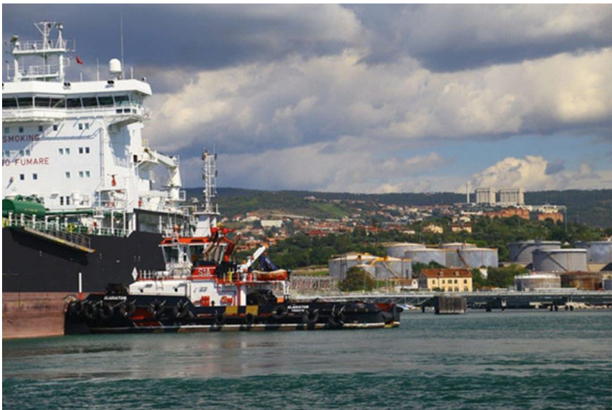
Fig. 5 Crude oil terminal in Trieste ( https://blog.omv.com/en/trieste-crude-oil-terminal-and-trans-alpine-pipeline/ )
