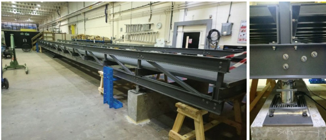
Fig. 16.1 Photograph of the FRP Bridge. Left. Full view of the structure. Right. Support conditions
