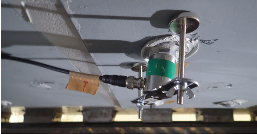
Fig. 11 AE sensors installation
