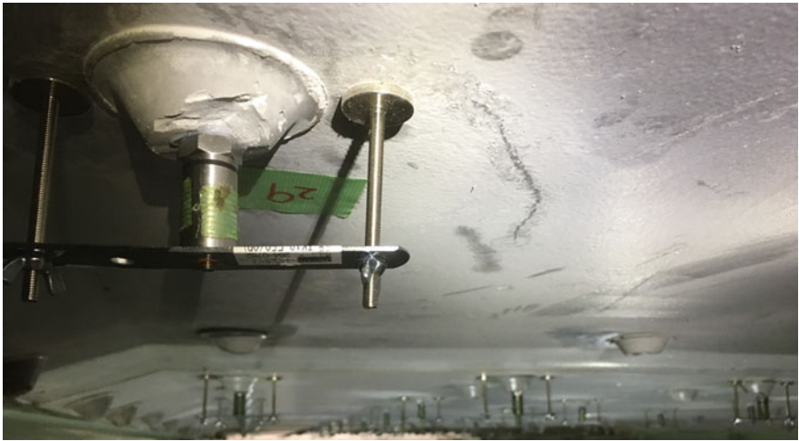
Fig. 3 The picture of sensors installation
