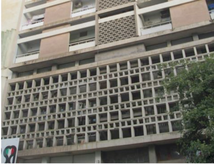
Fig. 6.17 Residential building in Maputo
