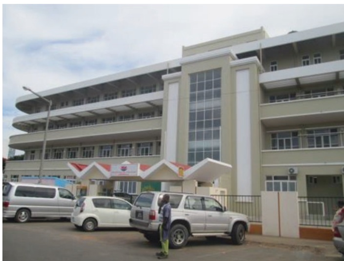
Fig. 6.21 Maputo Central Hospital: maternity wing
