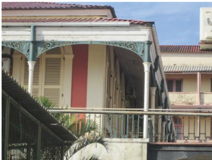
Fig. 6.2 Former offices of Delagoa Bay
