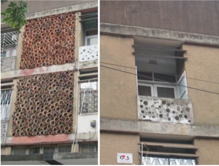
Fig. 6.29 The building for housing dockers
