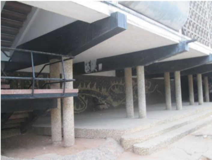
Fig. 6.28 Dragon House building
